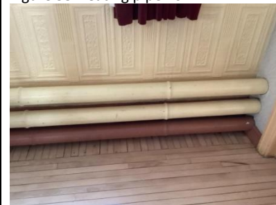
Figure 56 Distribution pipework
