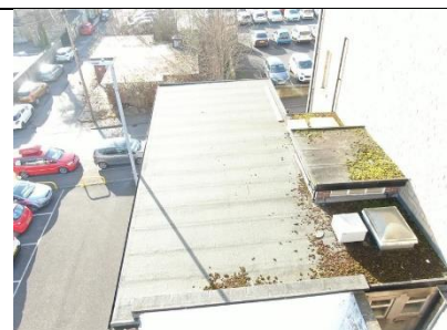
Figure 5 Rear felted flat roof
