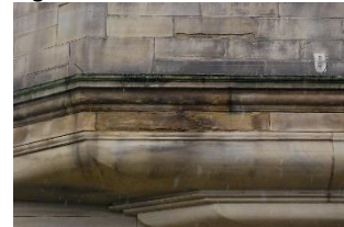
Figure 15 Typical area of repointing and descale
